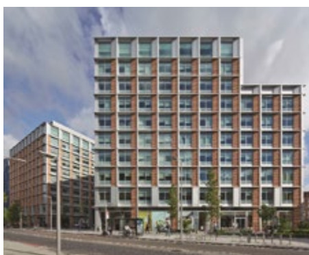
Bankside 2 & 3, London, United Kingdom, office building
