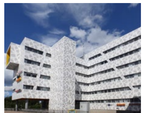
Safiiri, Espoo, Finland, office building
